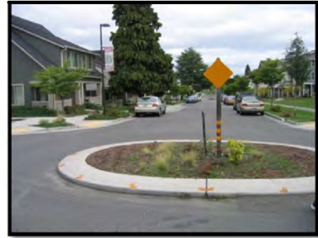
Photo 5.27: Traffic circle installed on a new residential street.
