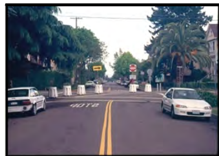
Photo 5.25: Diagonal diverter which still allows emergency vehicle access.
