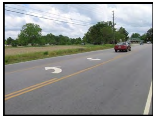
Photo 6.3: Two-way left-turn lanes remove turning vehicles from the main travel lane thereby reducing speed differentials and potential conflicts.
