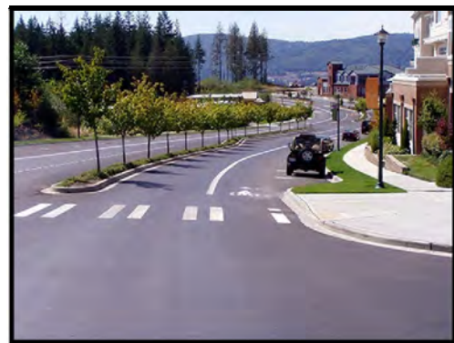
Photo 6.2: Raised median restricts access at desired locations.
