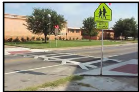
Photo 5.15: Raised crosswalk located near a school.
