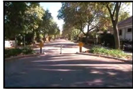
Photo 5.23: Full closure installed in a residential neighborhood.
