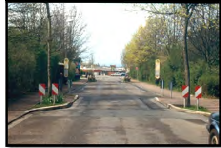
Photo 5.20: Choker installed to connect a trail at a midblock location.
