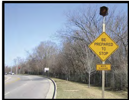
Photo 5.10: Advance warning sign for a traffic signal.
