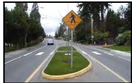
Photo 5.19: Refuge Island installed at a crosswalk.
