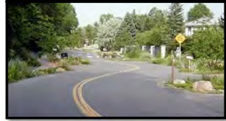
Photo 5.17: Chicane installed to force vehicle deflection.
