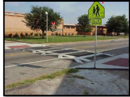
Photo 5.28: Raised Crosswalk installed near a school.
