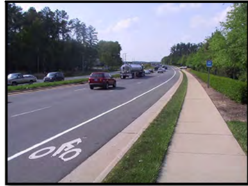
Photo 6.5: Complete street accommodating all users.
