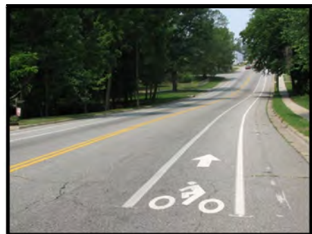
Photo 5.3: Pavement markings used to stripe a bike lane, creating a narrower travel lane.
