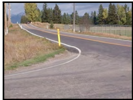
Photo 2.36: Hodgson Road / Whitefish Stage; from top to bottom: looking west; looking south; looking east; looking north.
