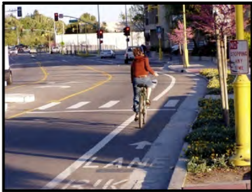
Photo 8.7: Bike lane installed along a three-lane roadway.
