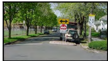
Photo 5.22: A half closure installed near a school.
