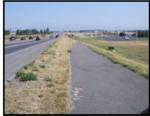
Photo 8.5: Shared-use path along US Highway 93.
